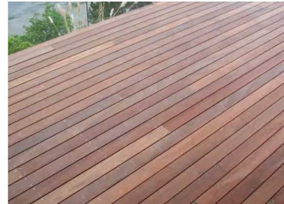
TIMBER DECKING ROOFTOP
